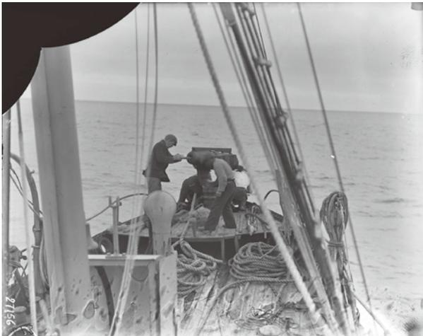
Loading the harpoon-gun. “The charge is 300 to 375 drams of very coarse, black powder which is… rammed home from the muzzle ; then come wads of okum (oakum の誤り), hard rubber or cork. After which the harpoon… is hammered solidly into place.”
